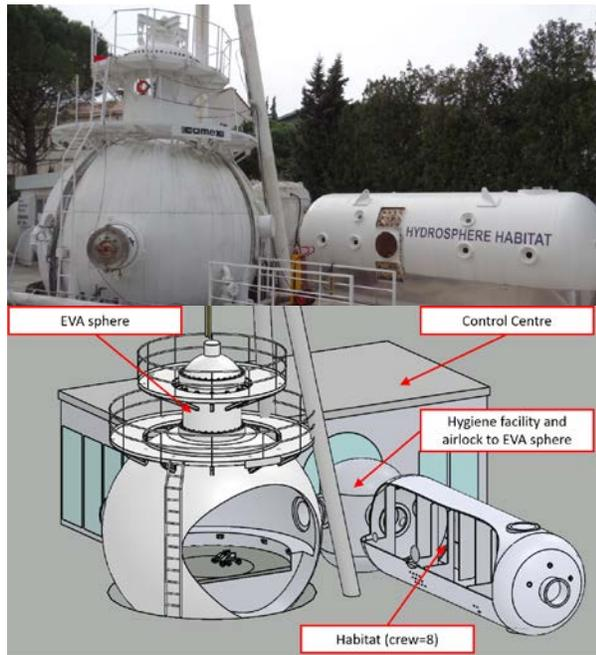
**Figure 4 Hydrosphere artificial analogue concept**
