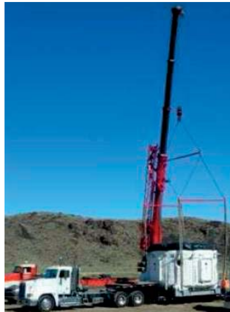
Figure 3: Unloading of the NASA HDU-PEM from the trailer.
